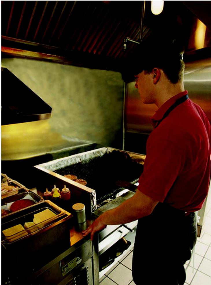
◀ *Slowing down hood fans during non-cooking periods saves energy, wear and tear on HVAC equipment, and reduces the entrainment of grease in the duct, among other benefits.*
