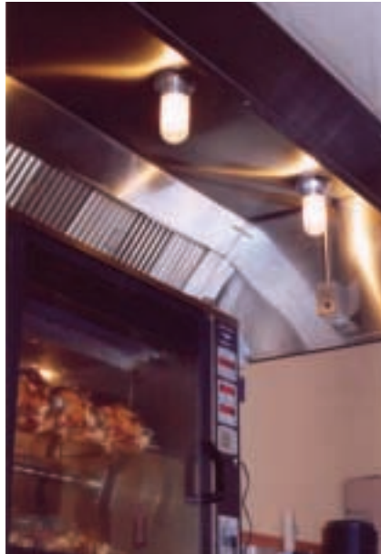
Optic sensors monitor when cooking is taking place. The fans then are ramped up accordingly until all effluent is removed from the exhaust-air stream.
